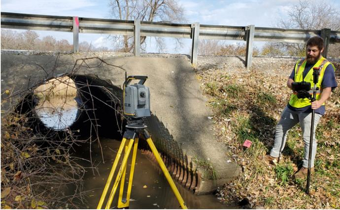
*Apprentice Ryan Baker of Hampton, Lenzini & Renwick, coding a topo point for a culvert relocation.*
