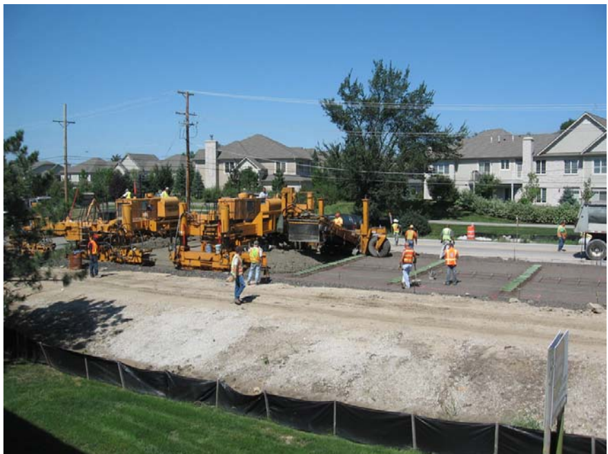
ILLINOIS ROUTE 22 DURING CONSTRUCTION
