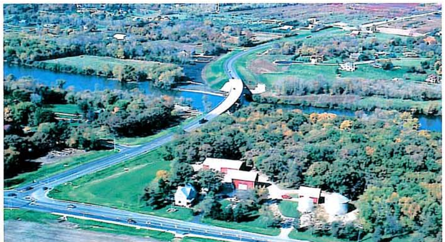
ORCHARD ROAD BRIDGE
